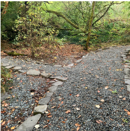
A freshly graveled and restored trail junction.
