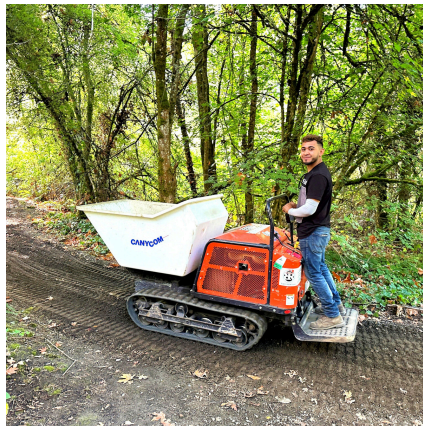
A dingo was required to move 130 tons of gravel to the trails.
